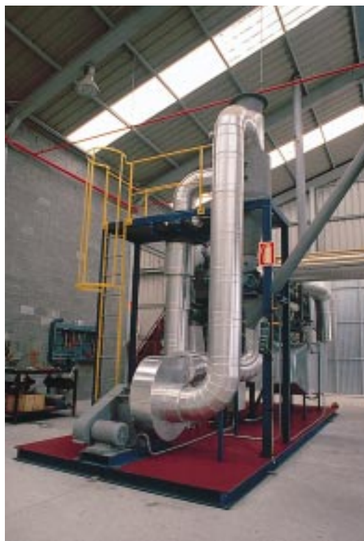
Figure 2: Pyrolysis pilot plant pretreatment area.
